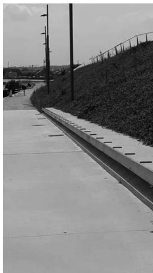
Fig. 4: Pig's ears deter unwanted skateboarding on concrete blocks in the Jardin du Musée des Confluences, Lyon (France). Photo: Smaniotto, 2018.
