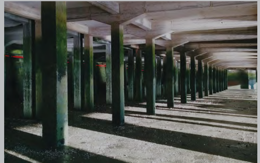
A fishing harbour located under a parking structure in Grandville, Normandy. September. 2018
