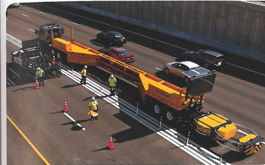
Illustration 6 - Mobile barrier in road work zone © www.mobilebarriers.com
