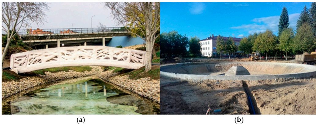
Figure 4. 3D printed infrastructure elements: (a) the first 3D printed bridge in Madrid (Spain) [11]; (b) restoration of the fountain in Palekh (Russia) [13].
