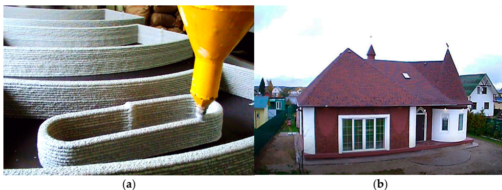
Figure 2. Printed house by a company AMT SPECALIA [7]: (a) printing process; (b) final product.
