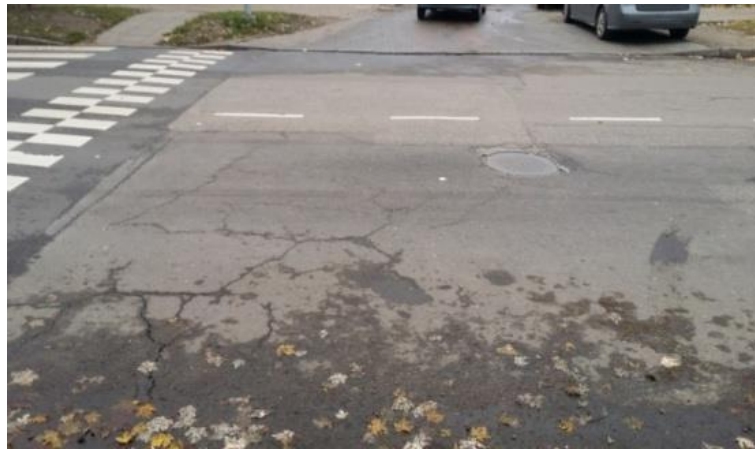
Fig. 3.17 Manhole near the speed table (Author's picture)
