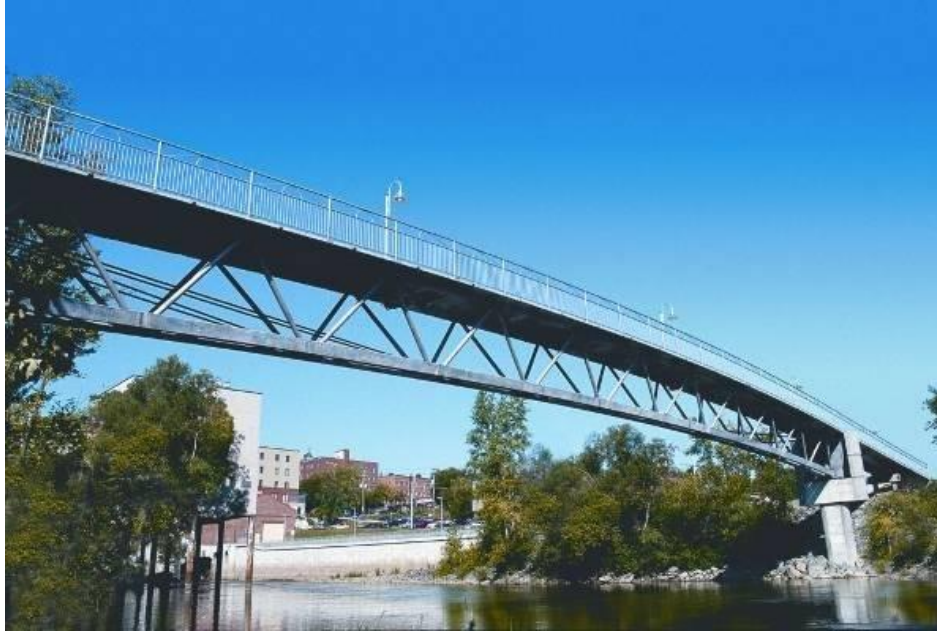
Figure 13 Sherbrooke Pedestrian Bridge
