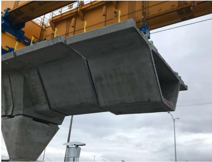
Figure 8 UHPFRC Bridge Girders
