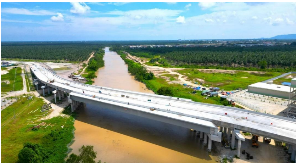
Figure 27 Langat River Bridge
