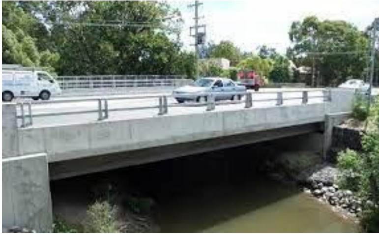
Figure 23 Shepherd Creek Bridge
