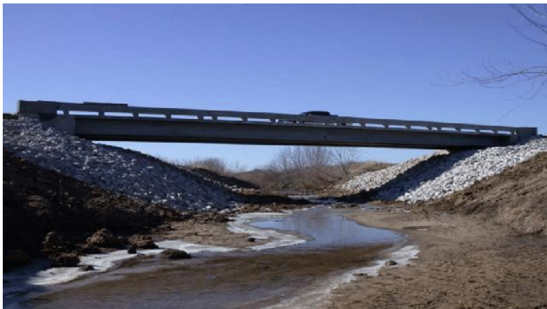
Figure 9 Mars Hill UHPC bridge in Wapello County, Iowa (sourced from Google)
