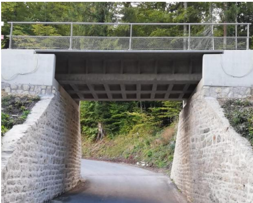
Figure 24 Aiguillon Railway Bridge
