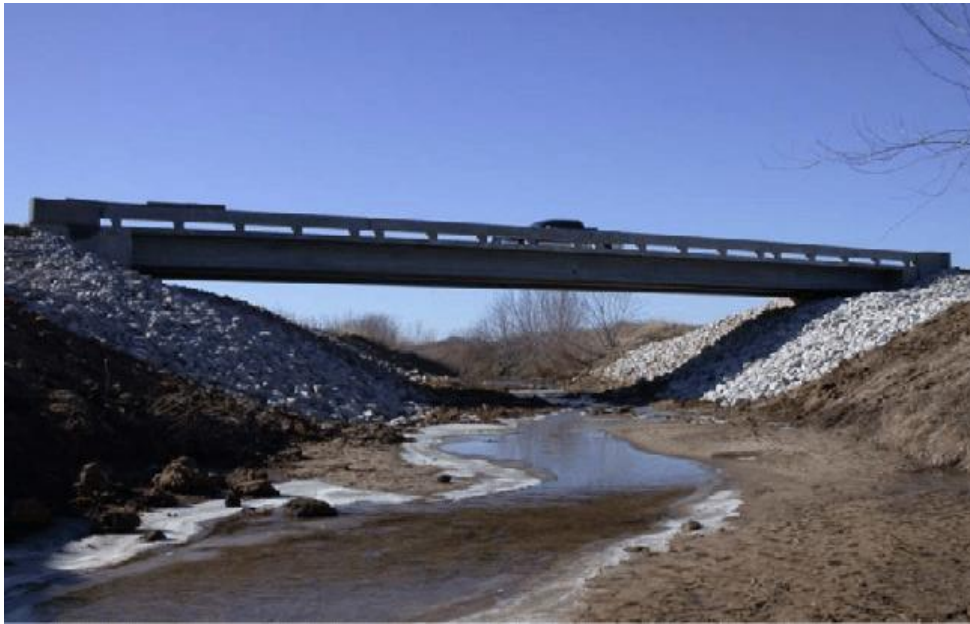
Figure 16 Mars Hill Bridge
