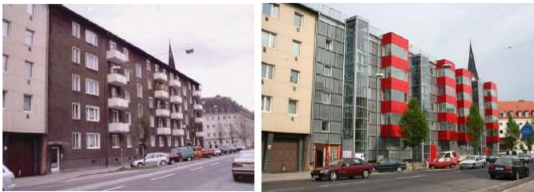
Figure 12. Building before and after renovation.
