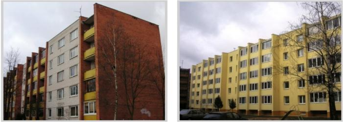
Figure 11. Building before and after renovation.
