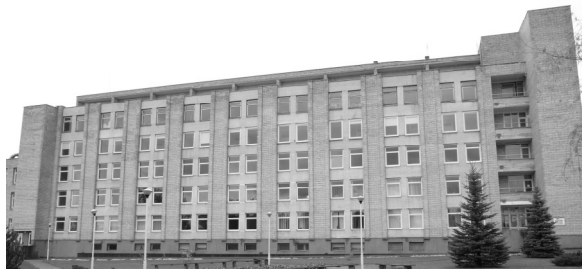
Fig. 3.6. The main building of the Kėdainiai hospital complex
