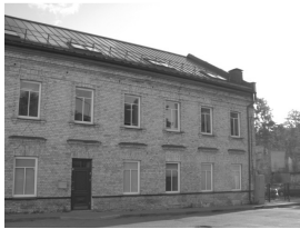
Alternative A (or a_1 ): a building in Pylimas street
