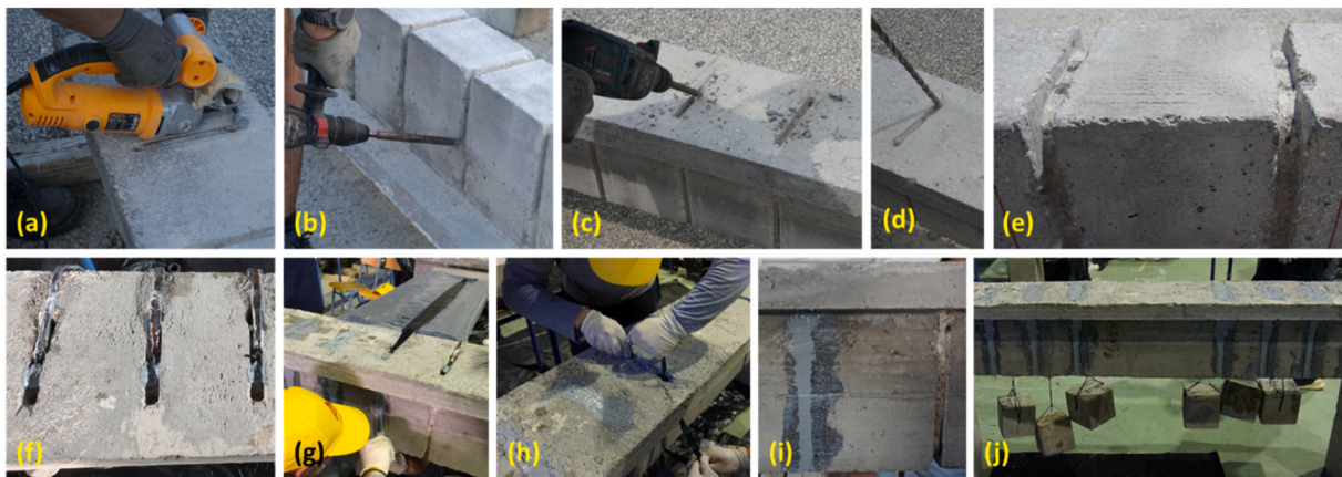
Fig. 7. Attaching NSM CFRP ropes: (a) creating notches; (b) and (c) ensuring the groove geometry by using a drilling machine; (d) drilling holes; (e) smoothing the web edges; (f) impregnation of small part of the rope end and placing it in the grooves of the upper part of the beam (slab); (g) prefilling the holes and grooves with epoxy resin to attach and impregnate the remaining rope; (h) placing the rope; (i) filling the resin; (j) stretching the rope with small weights.
