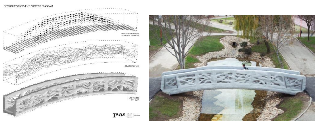
Fig. 1.5. Castilla-La Mancha 3D bridge (Buchanan & Gardner., 2021).
