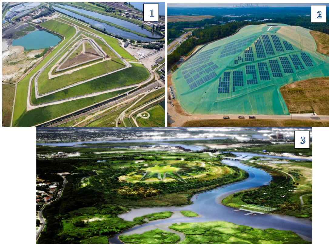
Fig. 1.24. Sustainable remediated landfills
