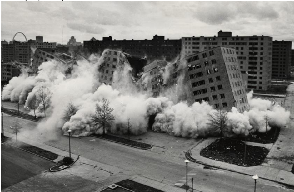
Fig. 6. The demolition of Pruitt-Igoe (© St. Louis Post-Dispatch)
