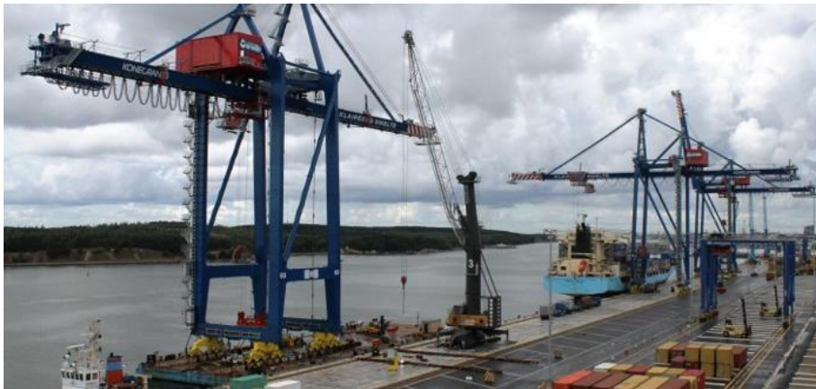
Figure 49. The photo of a STS crane in the container terminal area.
