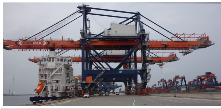
Figure 1. Quay crane in port of Rotterdam.
