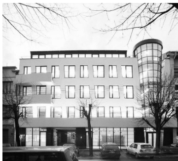
194 pav. Administracinis pastatas Kaune, archit. G. Natkevičius, V. Kuliešius, 2001 m. Fig. 194. Office building in Kaunas, by Architects G. Natkevičius, V. Kuliešius, 2001
