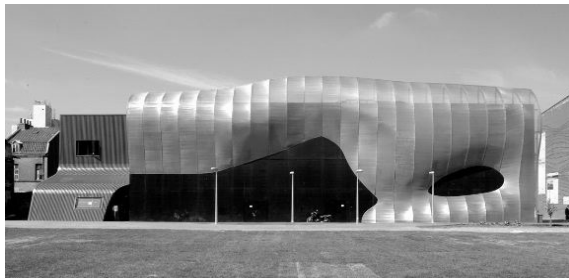
130 pav. Holoskin multifunkcinis pastatas Lilyje, Prancūzijoje, archit. L. Spuybroek, 2004 m. Fig. 130. Holoskin multifunctional building in Lille, France, by Architect L. Spuybroek, 2004
