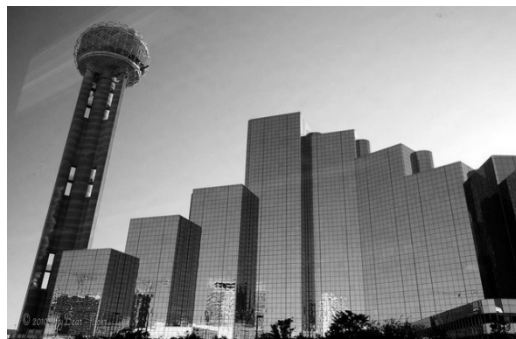
113 pav. Viešbutis Dalase, JAV, archit. W. Becket, 1976–1978 m. Fig. 113. Hotel in Dallas, USA, by Architect W. Becket, 1976–1978
