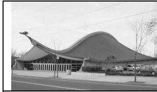
57 pav. Jeilio universiteto ledo ritulio arena Konektikute, JAV, archit. E. Saarinen, 1953–1959 m. Fig. 57. Ice hockey arena for Yale university in Connecticut, USA by Architect E. Saarinen, 1953–1959
